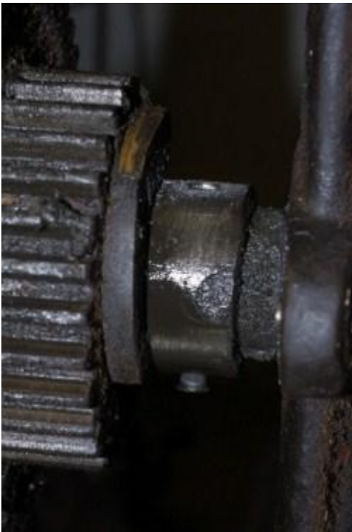
Pin partly tapped out from above
