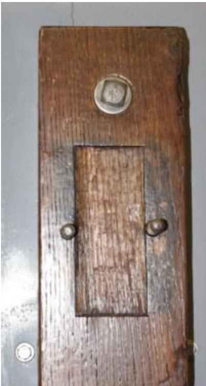
Original oak mounting board attached to new 4 x 10
