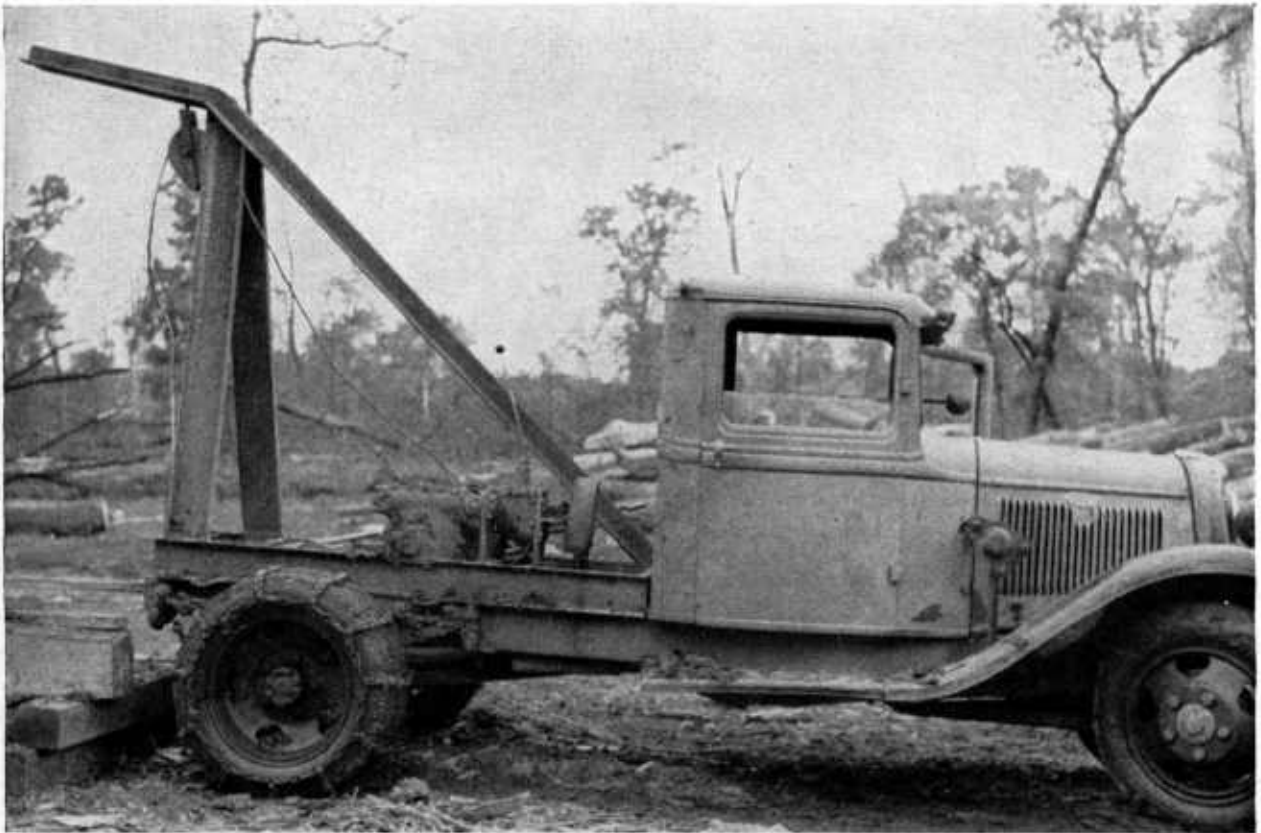
FIGURE 86.—Truck derrick for yarding logs.
