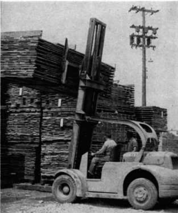
FIGURE 94.—Building a unit-package pile with a fork-lift truck.
