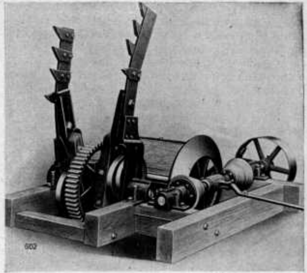
FIGURE 52.—Double-bar friction log turner.
