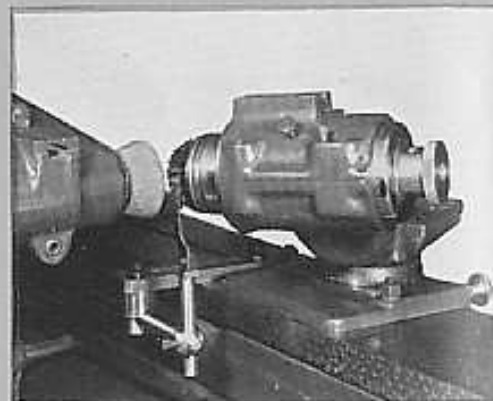
Grinding the teeth of an Angular Cutter
