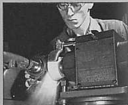
Grinding a spiral milling cutter
