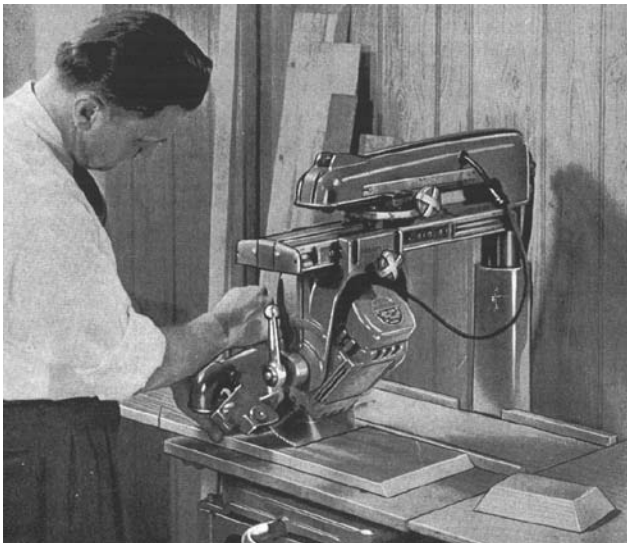
Figure 15. Multiplex 20-A radial arm saw, one of several Multiplex models that was manufactured at the Crescent factory under the Delta/Rockwell name beginning in 1950.
